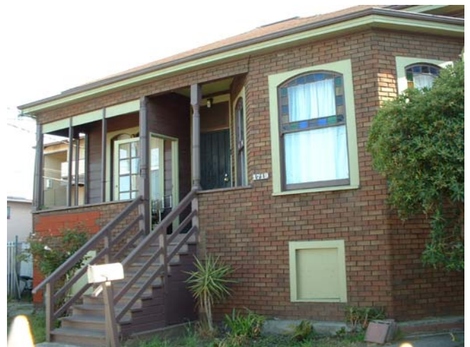
Luella’s house after Rebuilding Weekend
